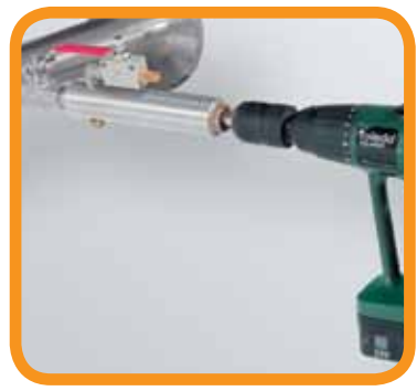
Drilling under pressure
